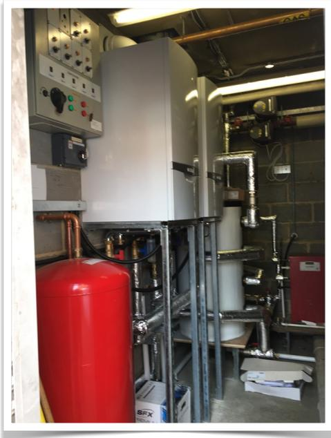
A condensing boiler captures much of the heat in the exhaust gas from a boiler and improves the efficiency by ~11%. Gas boilers can thus reach over 90% efficiency.
